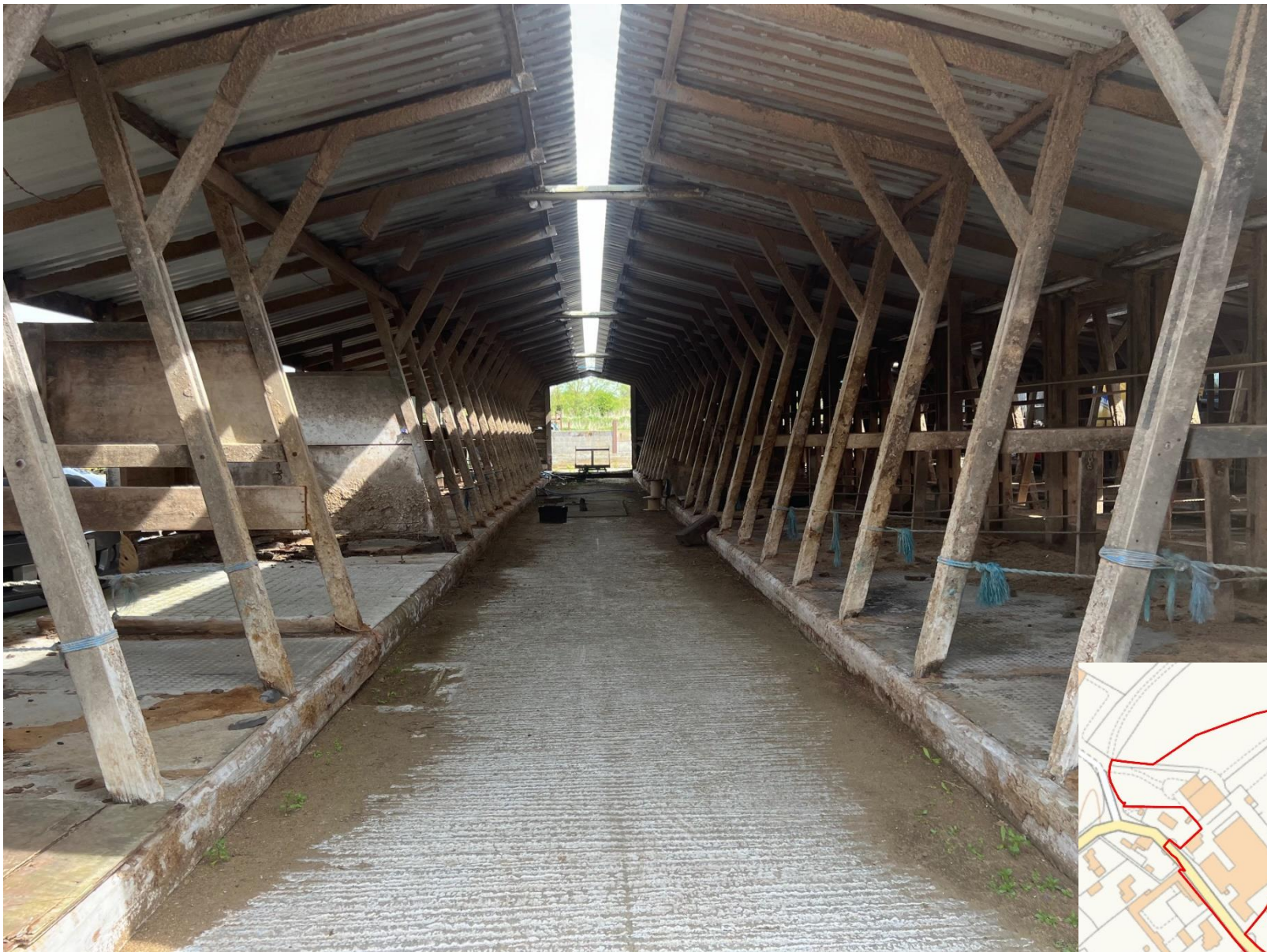
View within redundant barn
