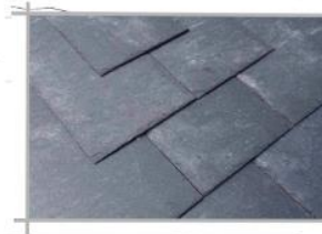
Typical natural slate for roof
