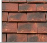
Suggested 'Wiltshire' blend of red-brown plain clay tiles for main roof.
